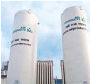
Air Products' LOX system for 1 st phase oxy-boost at Yongxin and now it serves as backup system to enhance 100% O 2 reliability
